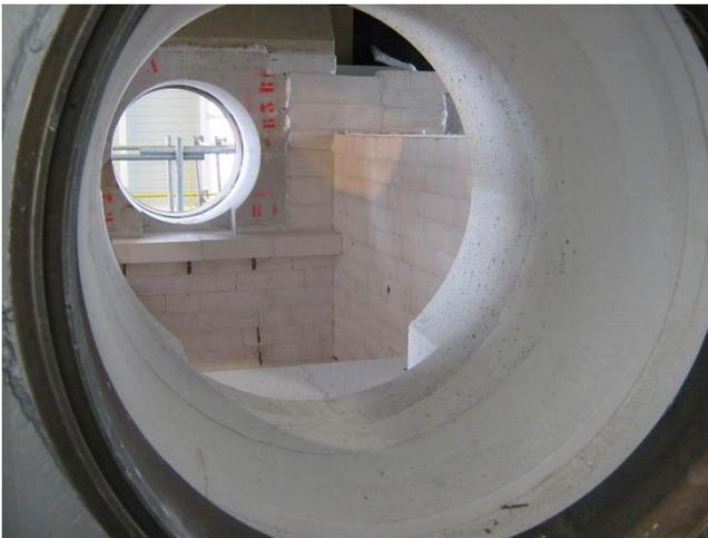
Vulcasil A99I is a +99% bubble alumina insulation material designed for use in reducing atmospheres such as hydrogen where the presence of silica is not permitted. Its resistance to hydrogen attack at high temperatures makes it ideal for use in bright annealing furnaces where Vulcan Refractories have unrivalled experience. Vulcasil HI 99 is also used as a backup lining in ammonia reformers and in areas where high purity insulation is required up to 1850°C.
