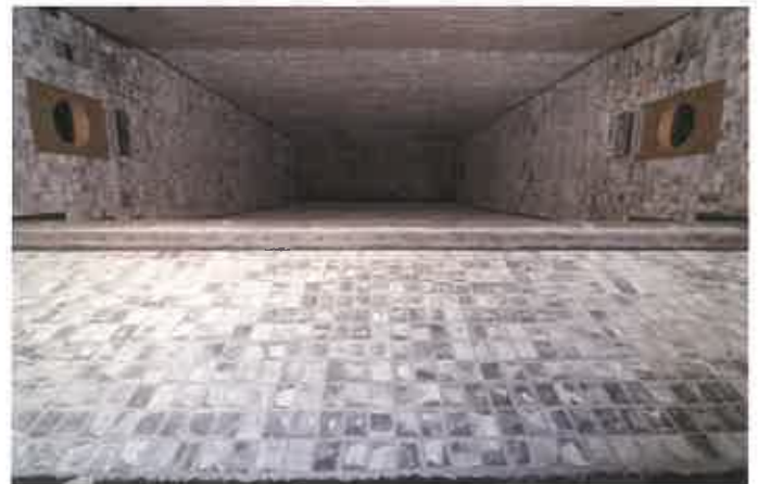
Silicon nitride bonded silicon carbide tiles freshly installed in an incinerator in mainland Europe
